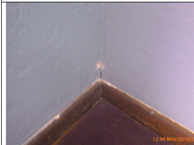
View of the ACM Heavy Mop Walls Sampling/Pastoral Staff (Photograph 11)
