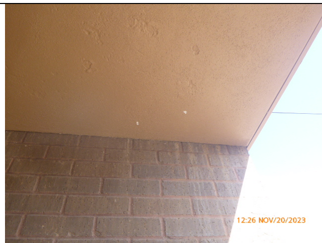
View of the Exterior Stucco (Photograph 18)
