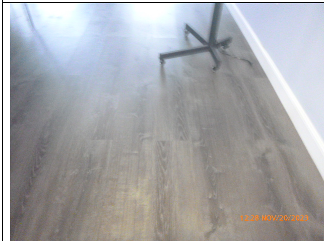
View of the Laminate Flooring (Photograph 11)
