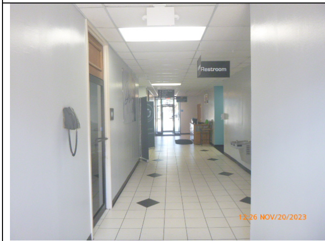
View of the Ceramic Floor Tiles and Walls in the Hallway (Photograph 03)
