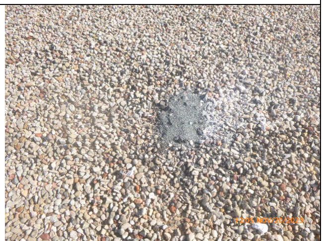
View of the Roof Core Sampling (Photograph 24)
