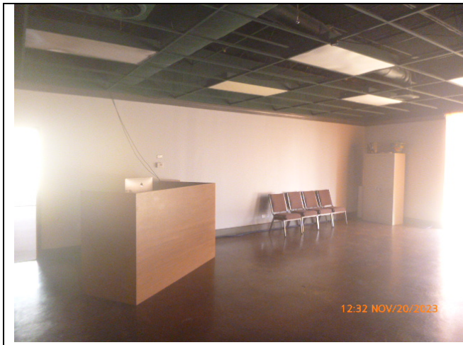
View of the ACM White Walls at the Student Room (Photograph 13)
