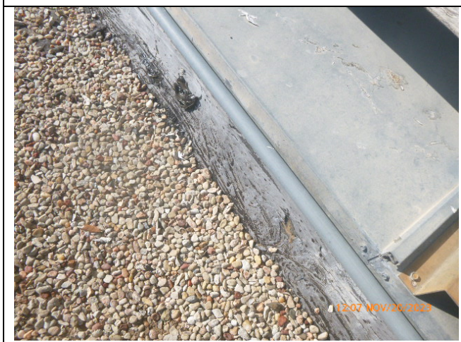
View of the ACM Roof Flashing Sampling (Photograph 23)
