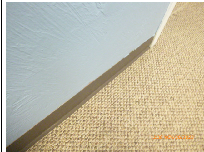
View of the Brown Cove Base (Photograph 17)
