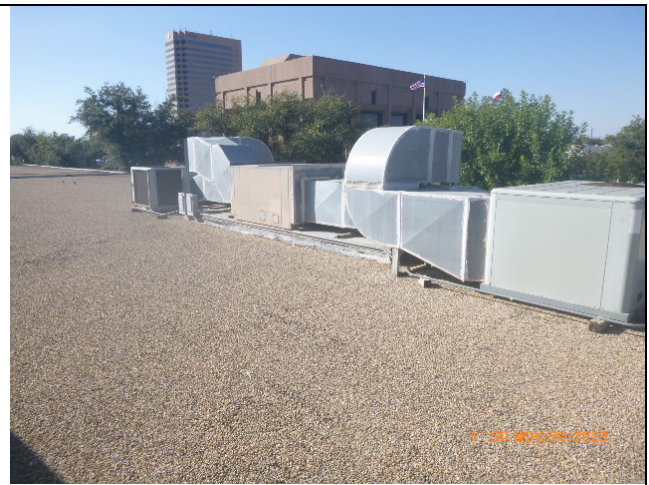
View of the Roof (Photograph 20)
