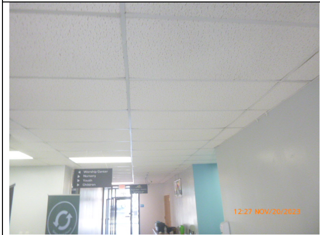
View of the 2'x4' Ceiling Tiles (Photograph 05)
