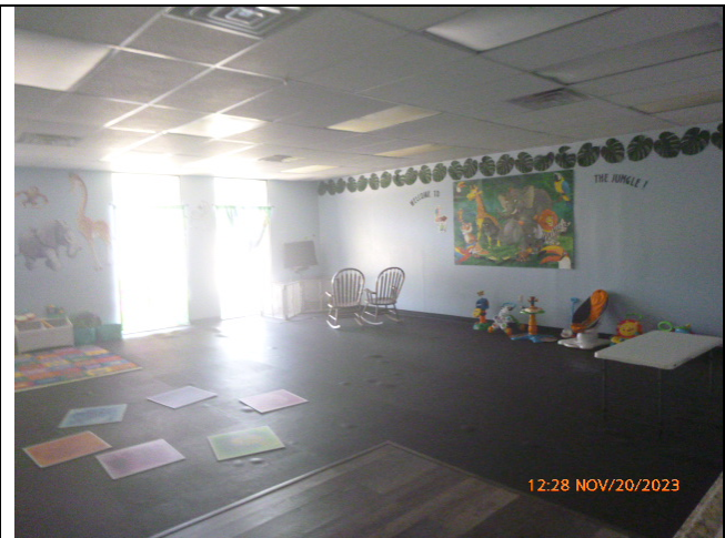
View of the ACM Dark Blue Walls (Photograph 08)
