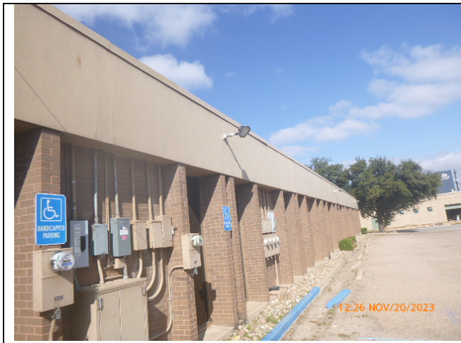
View of the Exterior Bricks (Photograph 19)
