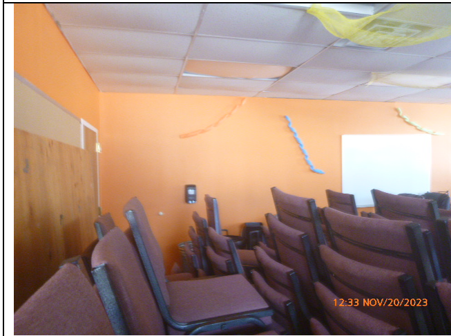
View of ACM Orange Walls at Room 16 (Photograph 15)
