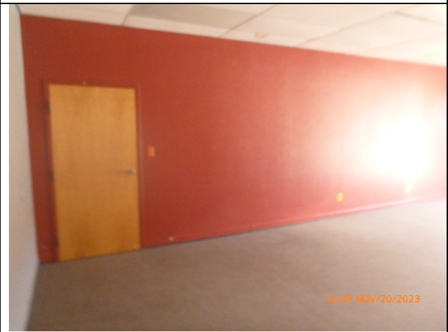
View of the ACM Orange Walls (Photograph 10)
